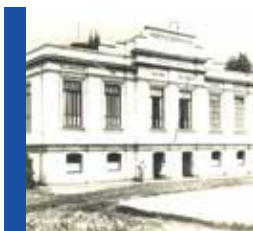
Hospital São Geraldo – HC/UFMG, Belo Horizonte
