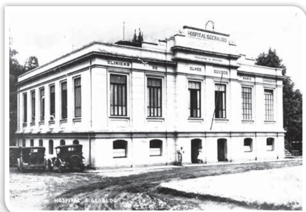
HOSPITAL SÃO GERALDO – HC/UFMG, BELO HORIZONTE
